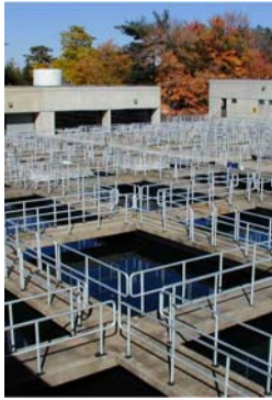
Andover's Water Treatment Plant—Sedimentation Basins
