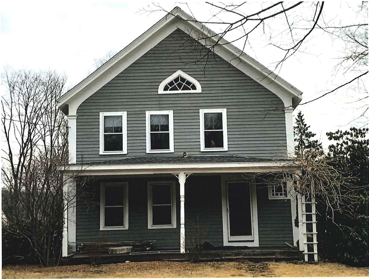
Photo 3, West Elevation, March, 2020
