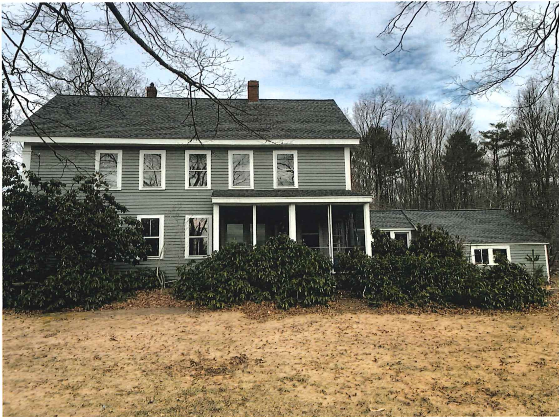
Photo 5, South Elevation, March, 2020
