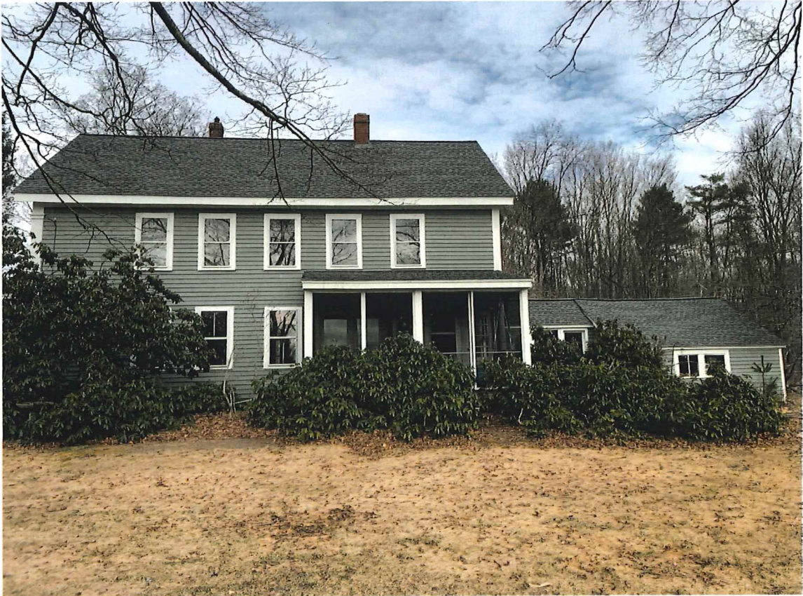
Photo 5, South Elevation, March, 2020
