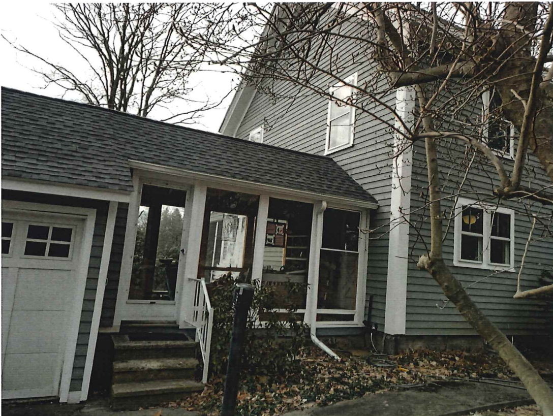
Photo 10, North Ell detail, March, 2020
