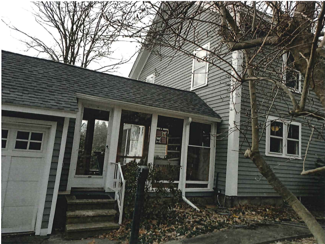
Photo 10, North Ell detail, March, 2020
