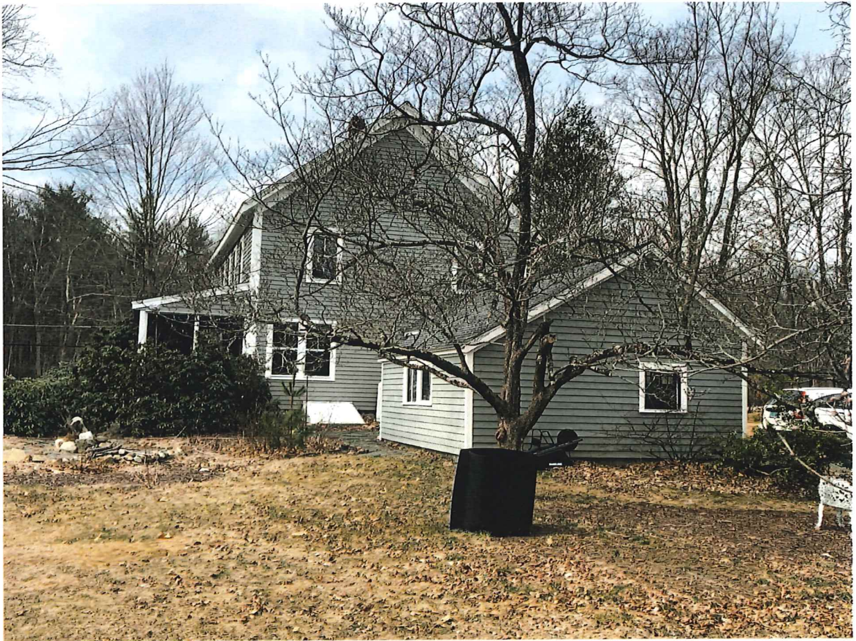
Photo 7, South & East Elevation, March 2020
