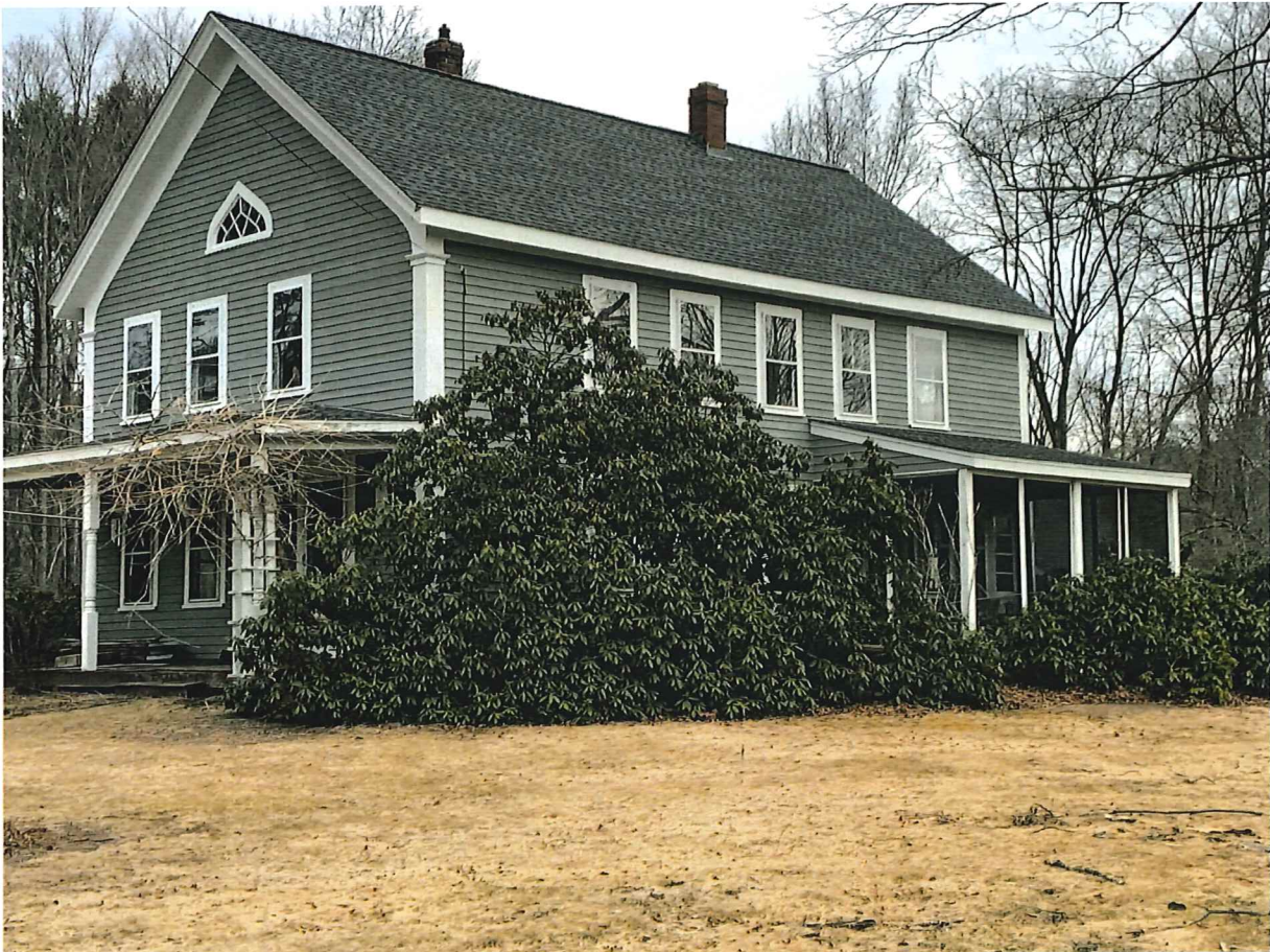
Photo 4, West & South Elevation, March 2020
