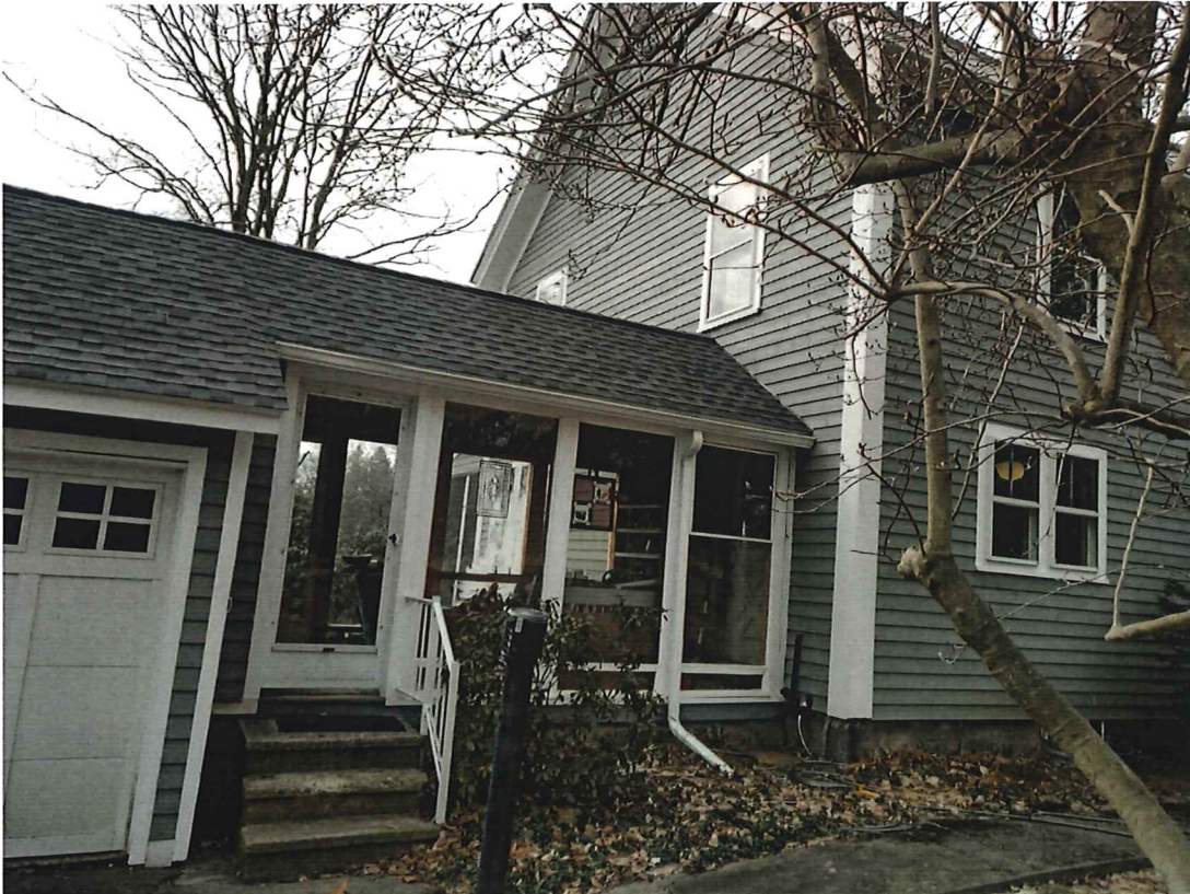
Photo 10, North Ell detail, March, 2020
