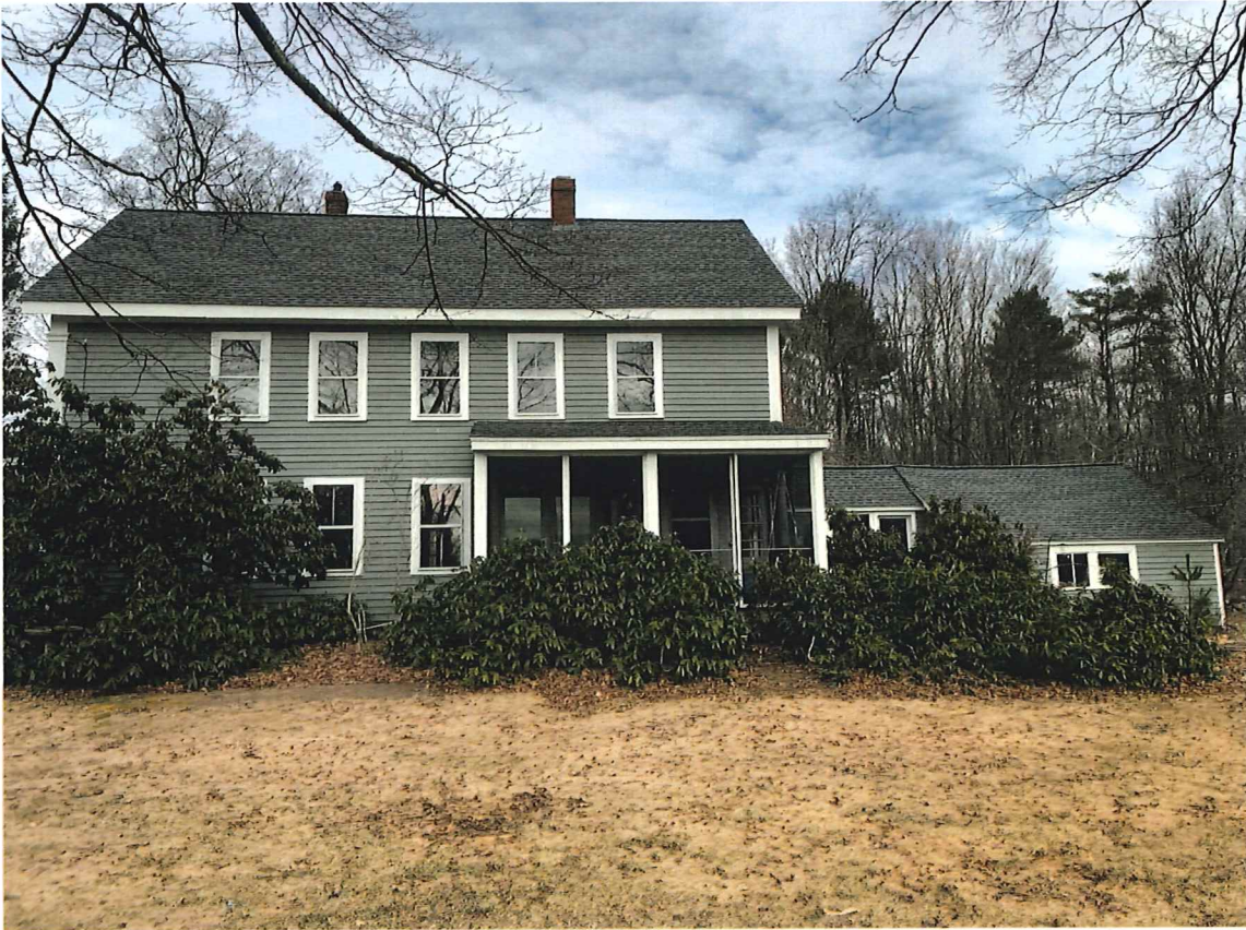
Photo 5, South Elevation, March, 2020
