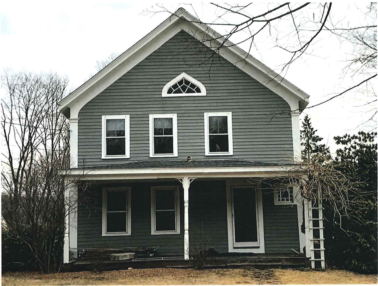
Photo 3, West Elevation, March, 2020
