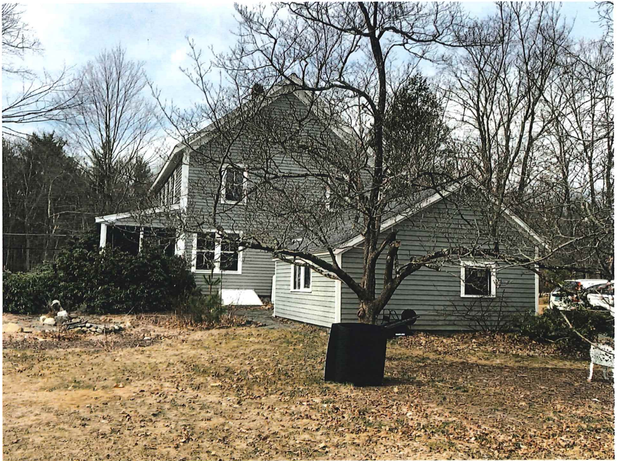
Photo 7, South & East Elevation, March 2020
