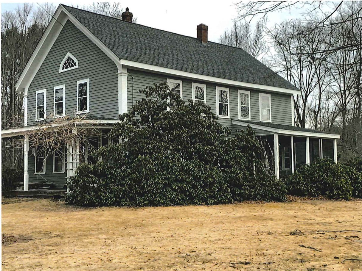
Photo 4, West & South Elevation, March 2020
