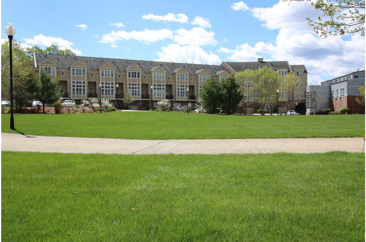
Figure 11 Powder Mill Square
