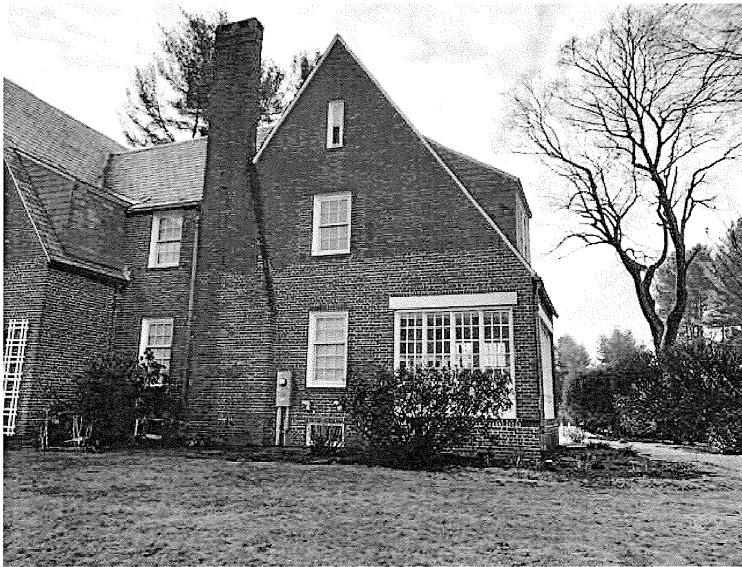
Photo 5 North Elevation Detail 1-15-2021
