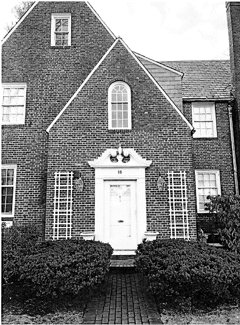
Photo 4 North Elevation Entry 1-15-2021
