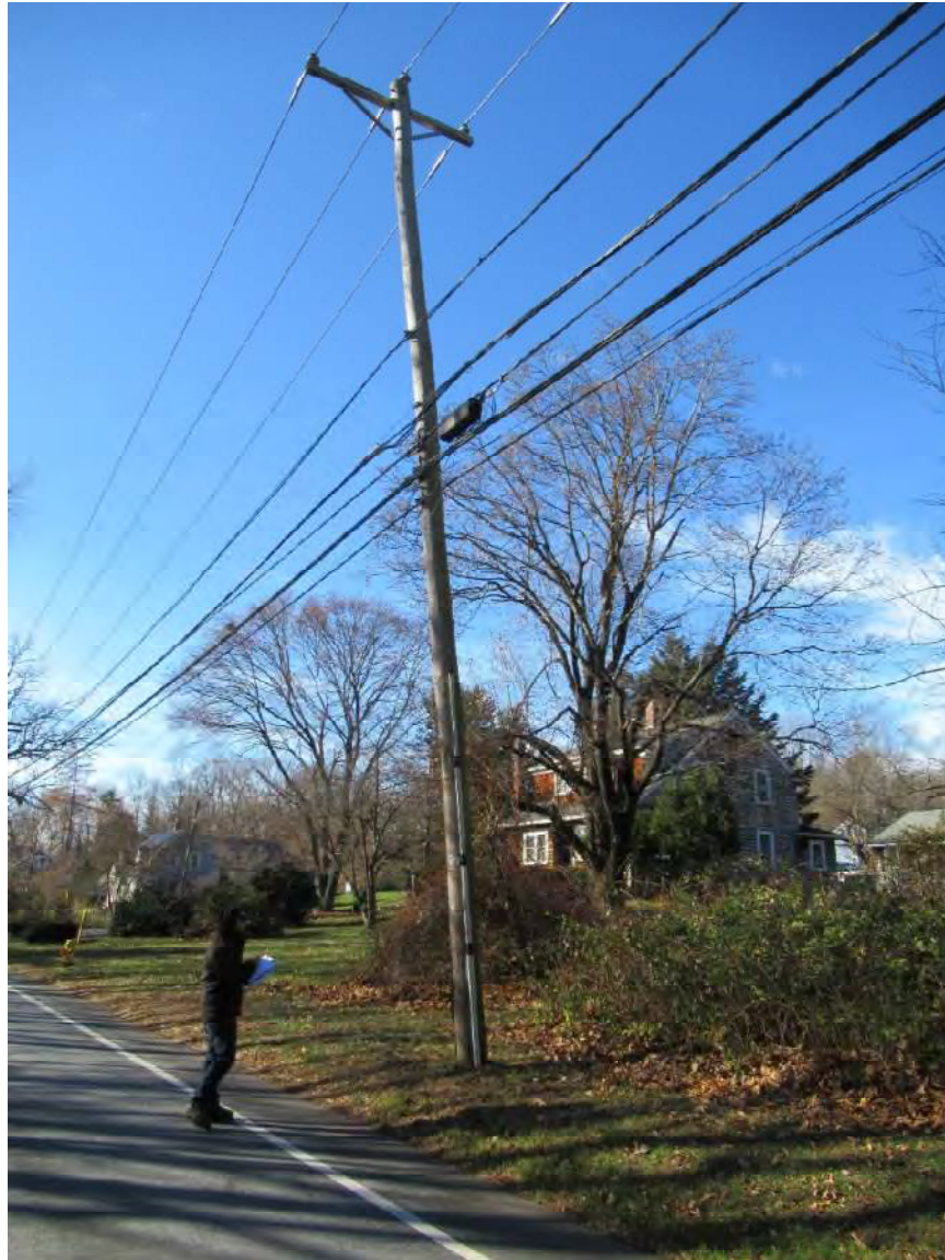
Photo 1: Sample photo illustrating the existing wood pole.
