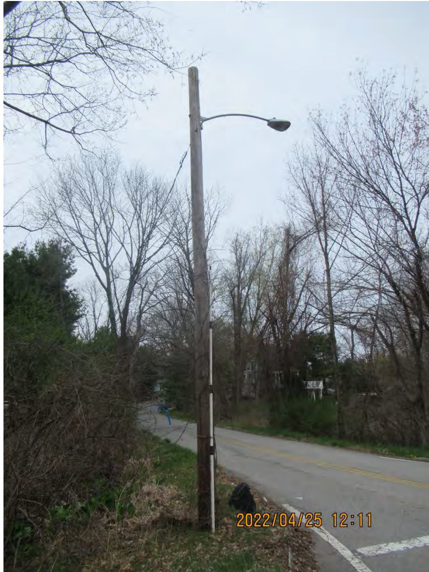
Photo 1: Sample photo illustrating the existing wood pole.
