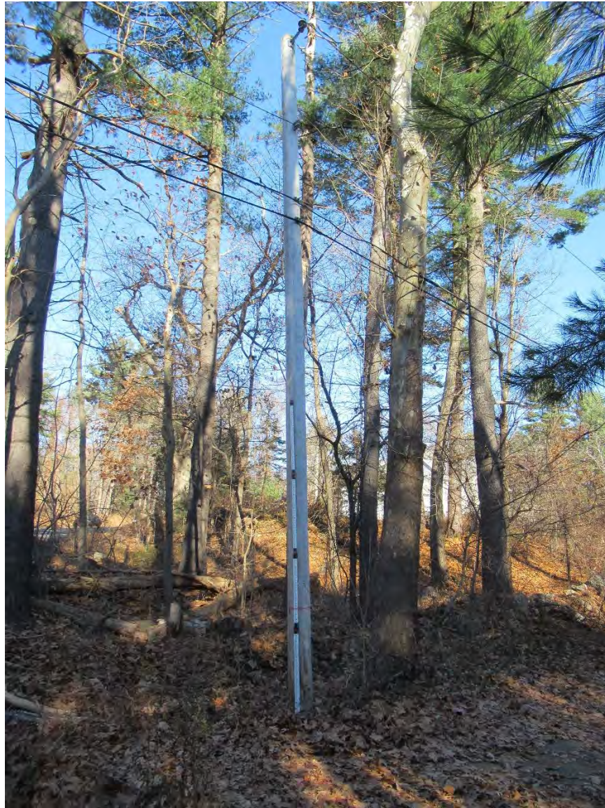
Photo 1: Sample photo illustrating the existing wood pole.
