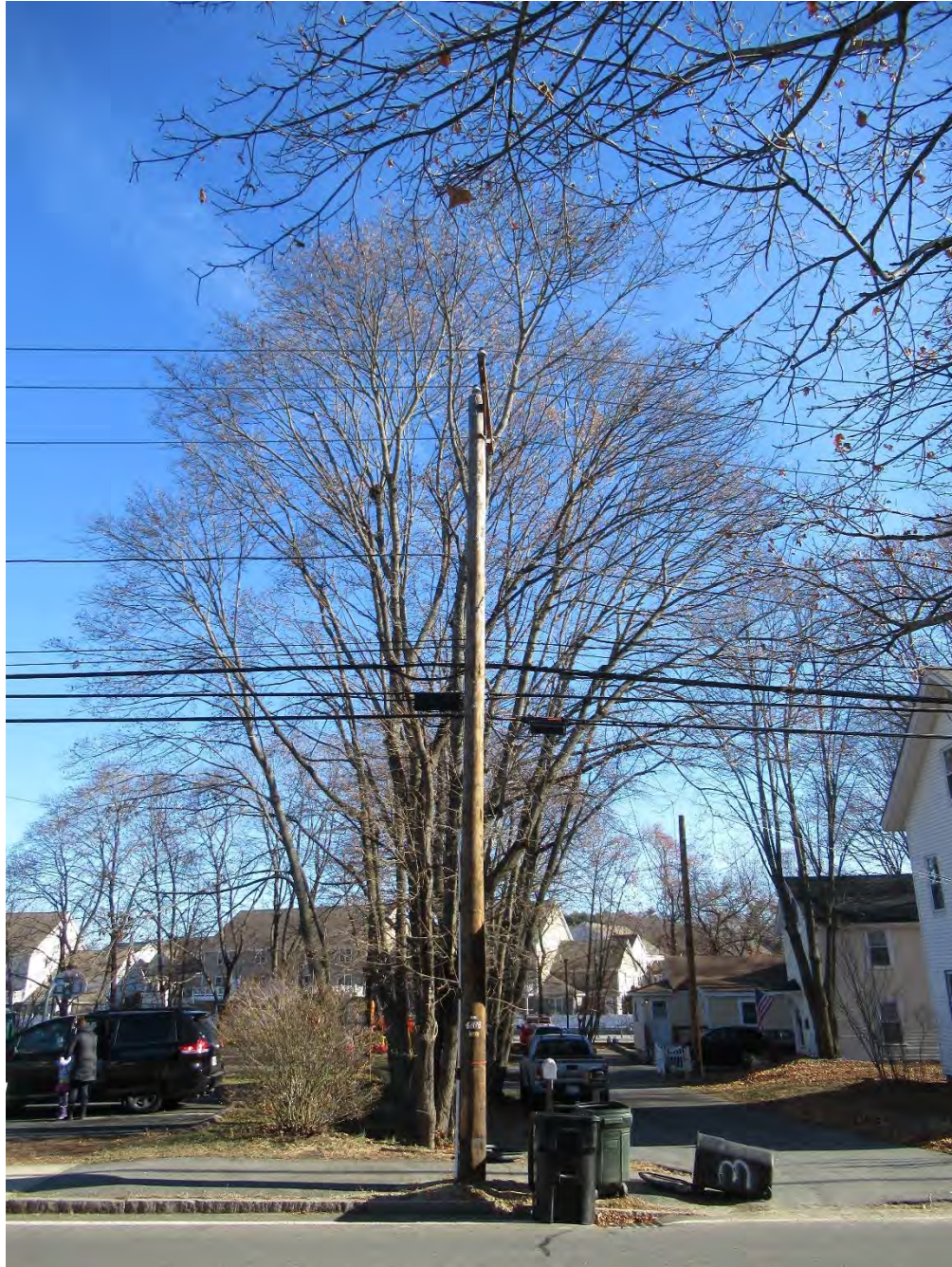
Photo 1: Sample photo illustrating the existing wood pole.
