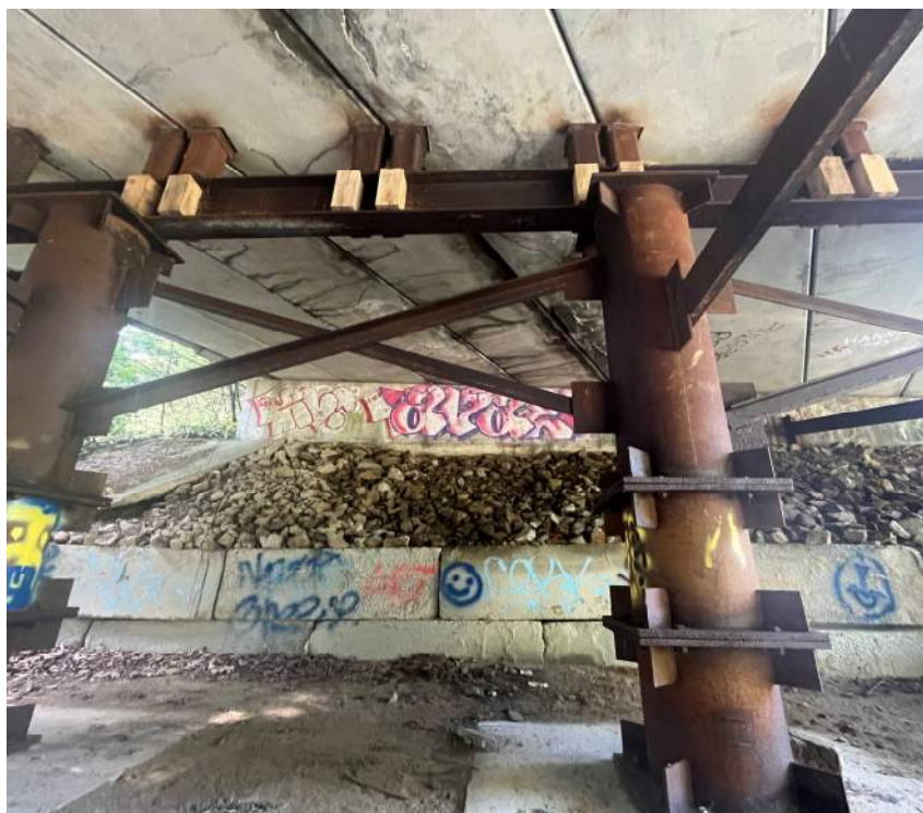
Shoring Towers in Place
