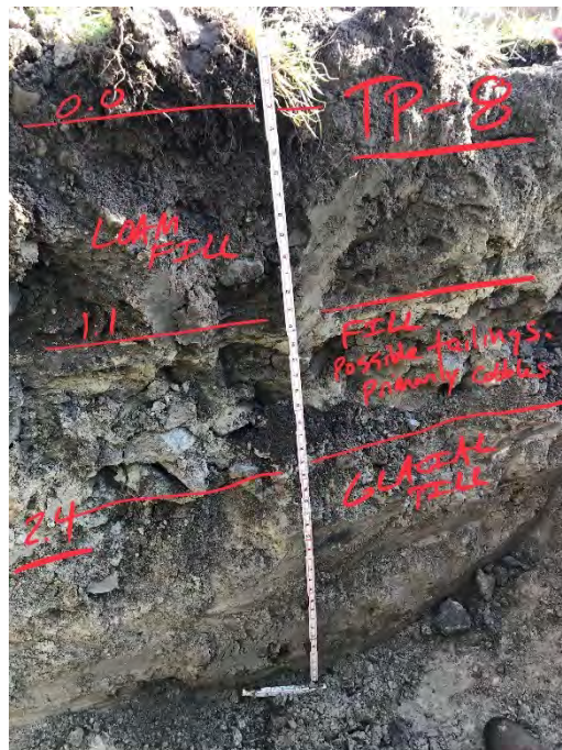
Photo 16: View of the sidewall at test pit HA21-TP8, showing soil stratigraphy. Top of Glacial Till was encountered at approximately 2.4ft bgs and is underlying loam and cobble Fill layers.
