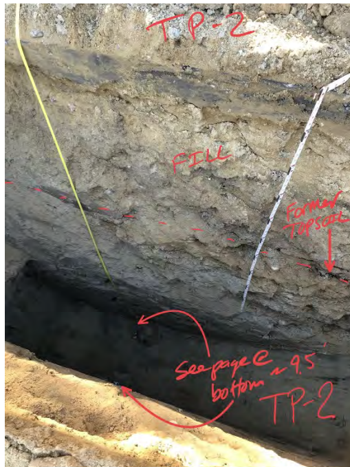
Photo 4: Test pit HA21-TP2. Former Topsoil layer observed in the Fill at the interface with the underlying Glacial soils. Water seepage observed at approximately 9.5 ft bgs.
