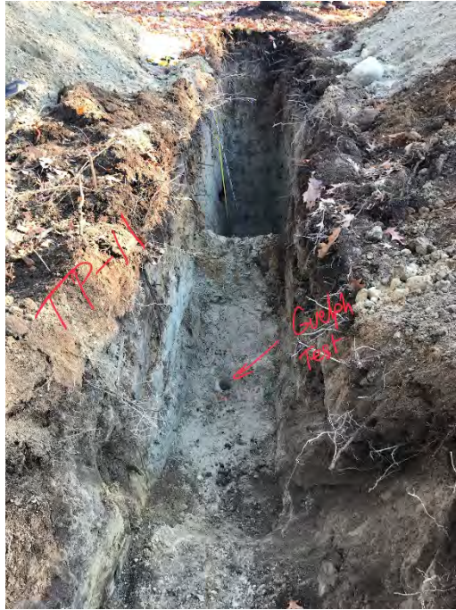
Photo 19: Guelph permeameter test conducted at test pit HA21-TP11.
