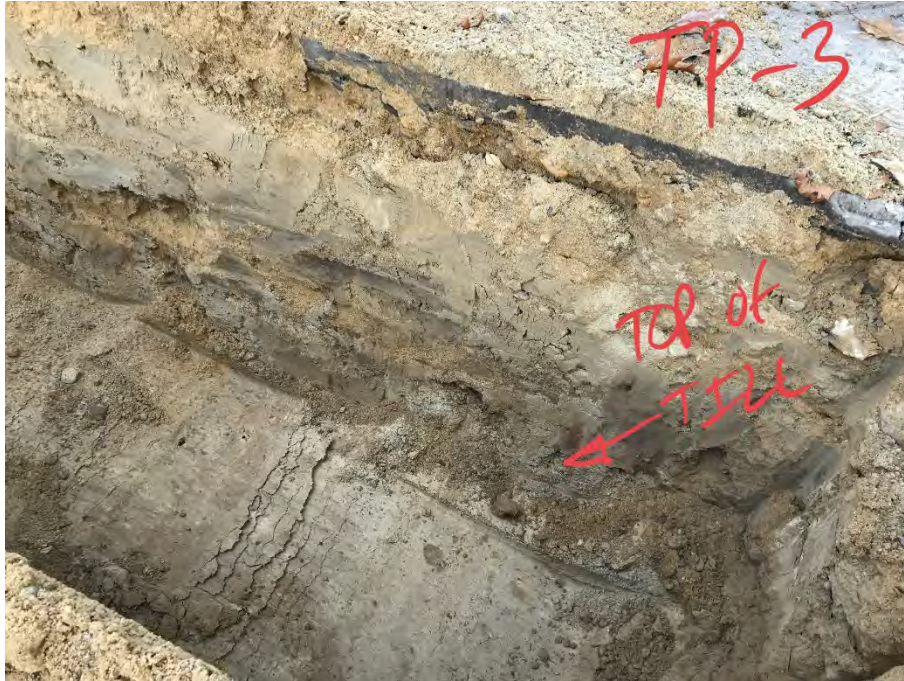
Photo 7: Completed excavation at test pit HA21-TP3. The top of the Glacial Till deposit is called out in the photo.
