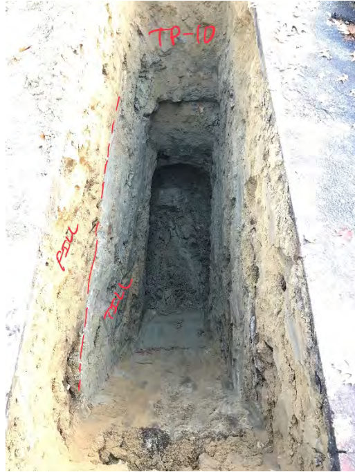
Photo 17: Completed excavation for test pit HA21-TP10.
