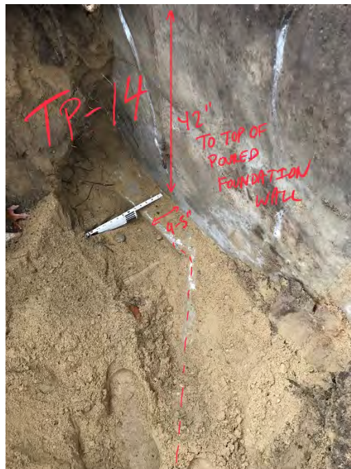
Photo 26: Close-up view of building foundation within test pit HA21-TP14.
