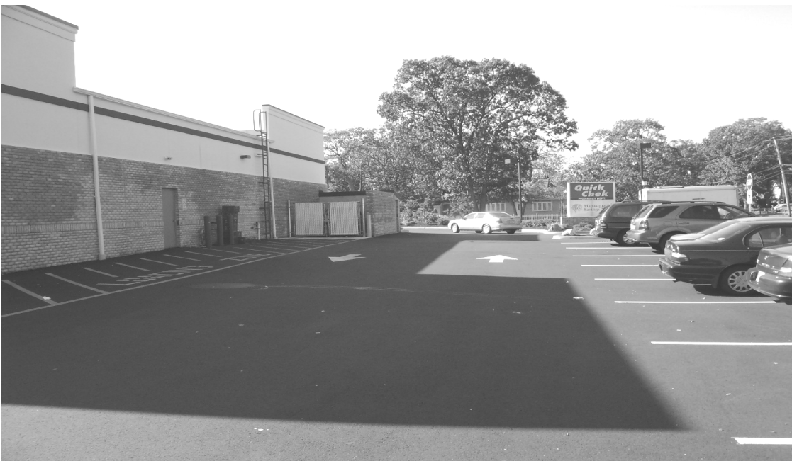
Figure 5 View of back parking lot area of Manasquan Savings Bank study site
