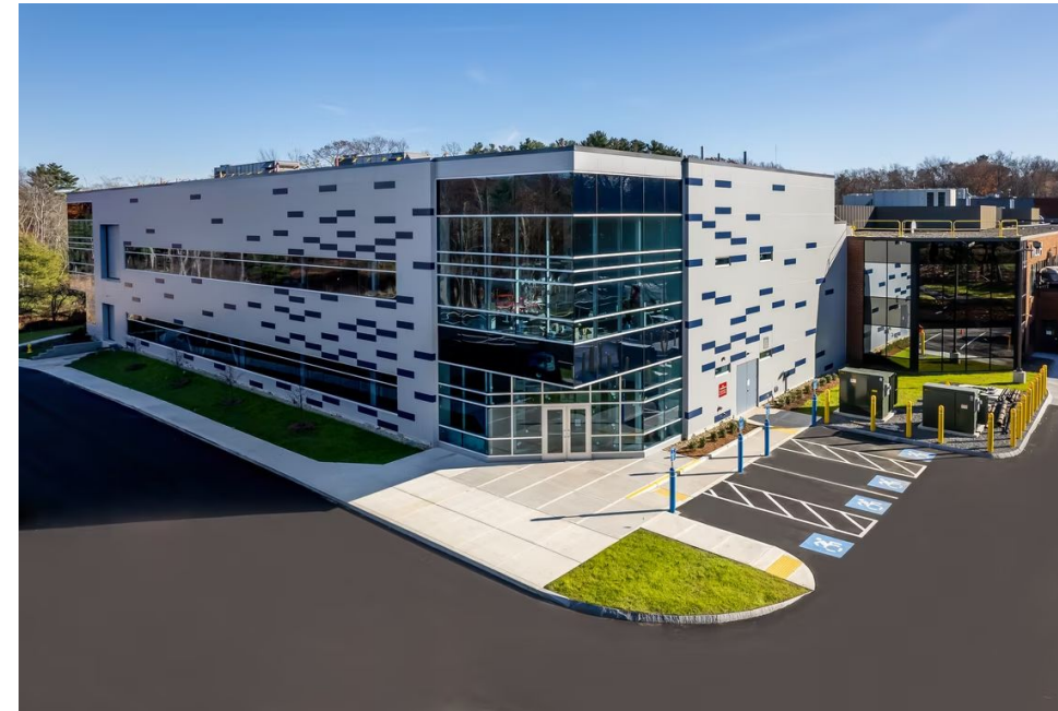
Andover's new Vicor CHiP fabrication plant, opened in 2022
