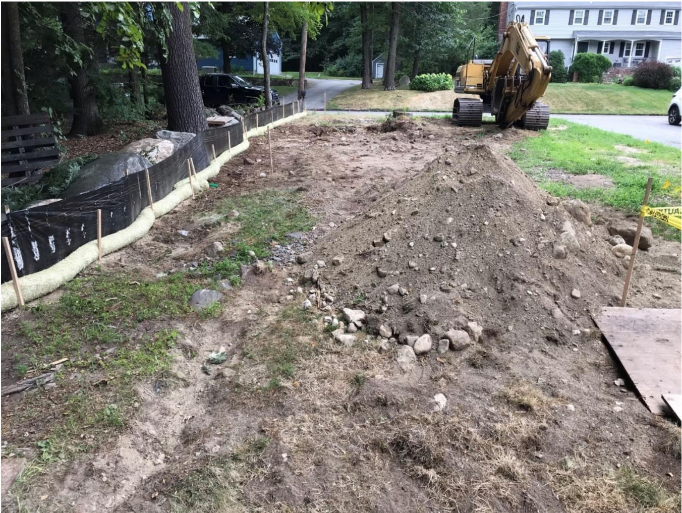
Picture 1. Straw wattles – along with black silt fence - staked in place at the limits of work of a septic system replacement project on the property of a single-family home in Andover. When used in conjunction with silt fence, straw wattles are placed in front of the silt fence to capture runoff, soils, etc. before they migrate off of a worksite.
