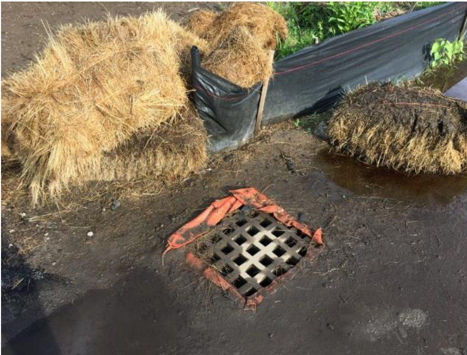
Picture 11. Silt sack in place during a construction project in Andover. Note evidence of silty/muddy water around catch basin and efforts to protect catch basin with hay bales and silt fence.
