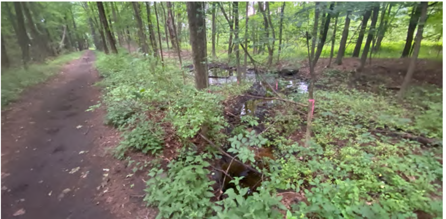
Photo #4: View of a stream crossing and existing culvert, looking north-northeast.
