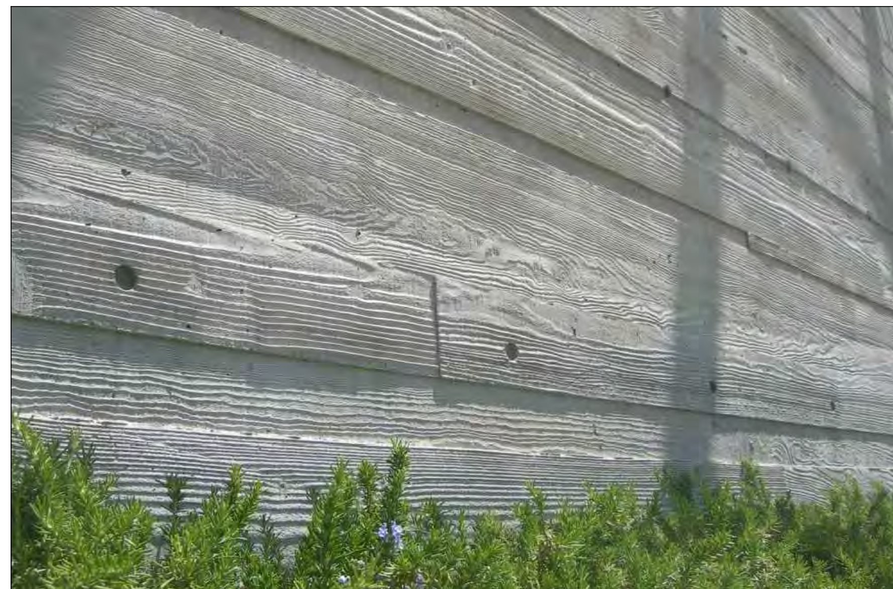
6 BOARD FORM CONCRETE FINISH NTS
