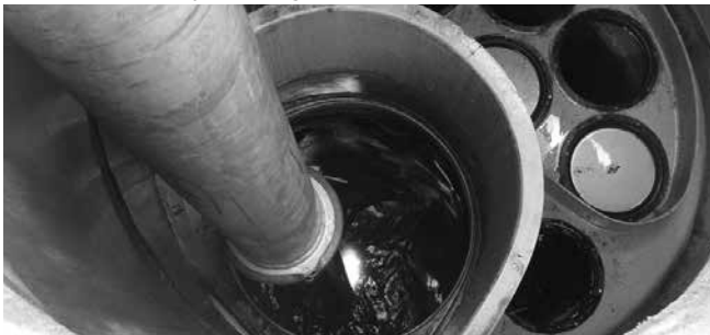
Vacuuming Sump Through MAW
