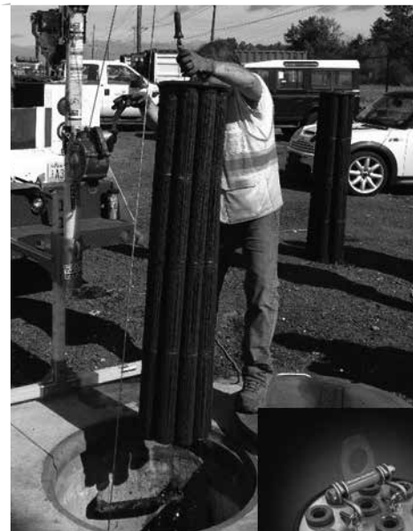
Cartridge Removal & Lifting Device
