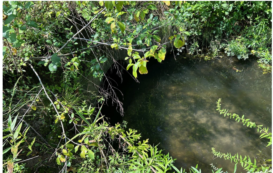
Typical views of existing conditions at the existing 48-inch diameter culvert (no evidence of erosion from scouring).
