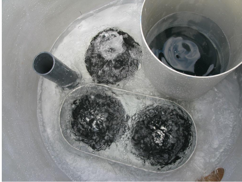
Figure 8 Top view photo of the Jellyfish Filter JF4-2-1 during operation. Filtered water exits the cartridge lid orifice as a pulsating fountain.
