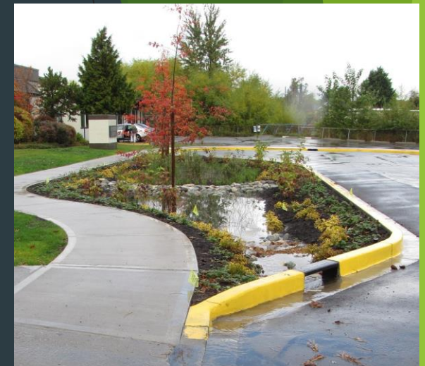
Bump-outs (also consider bump-outs where sidewalk section abuts low-speed road so that tree can access ROW and front lawn space without sidewalk between?)
