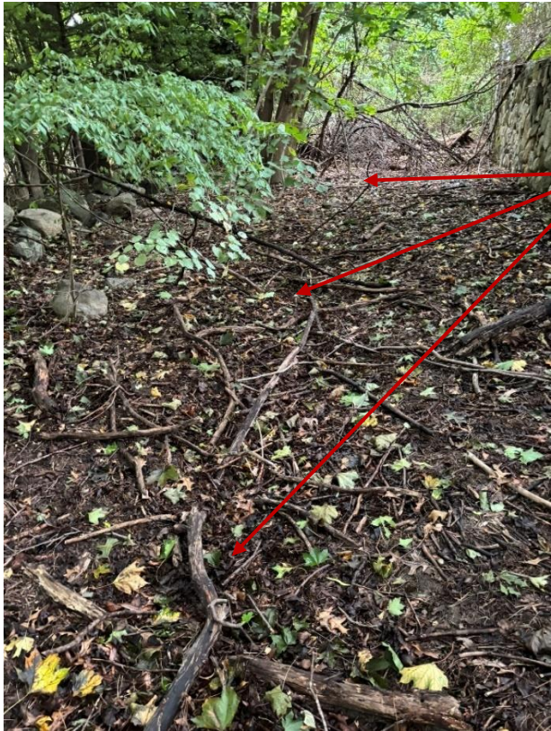
Man-made swale that directs stormwater into the catch basins on the Bancroft School Property. Please note the stone retaining wall in the background.
