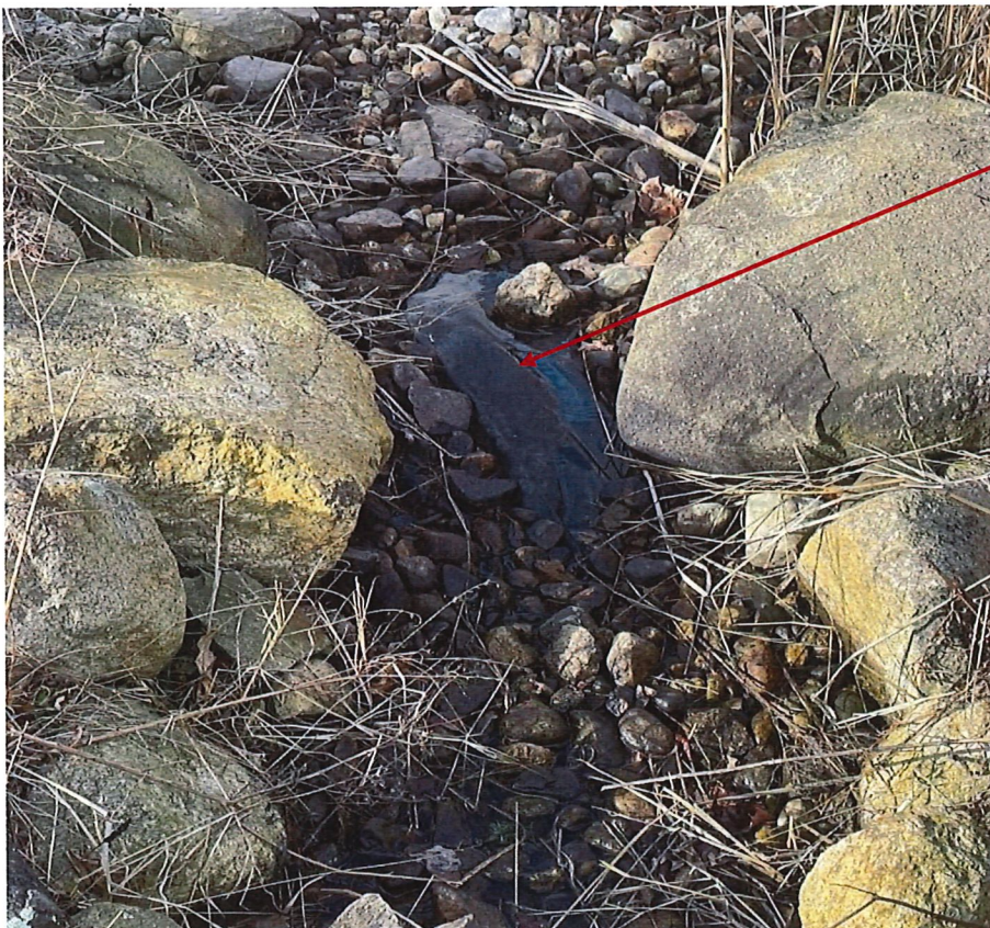
Landscape stream with rubber barrier liner.
