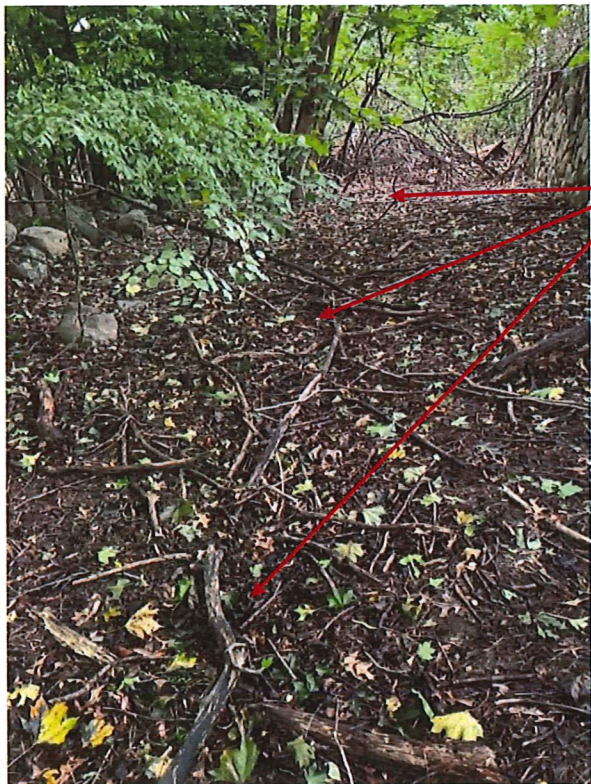
Man-made swale that directs stormwater into the catch basins on the Bancroft School Property. Please note the stone retaining wall in the background.
