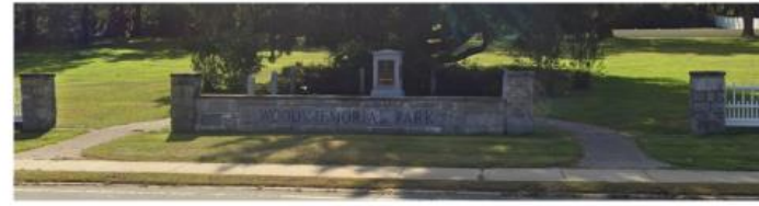
WOOD MEMORIAL PARK STONE WALL, PILLARS AND FENCING
