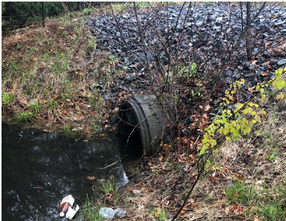
Figure 3 – infiltration basin outlet pipe flowing freely, no sedimentation visible
