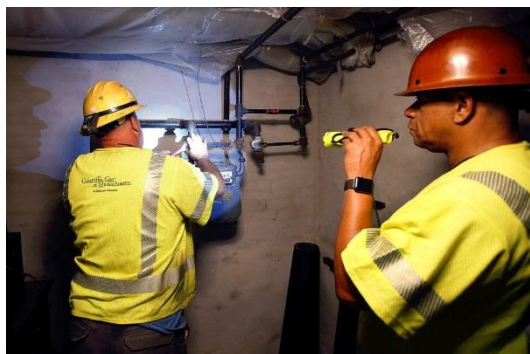
Figure 18: Render-Safe Teams Access the Interior of a Structure to Inspect the Gas Meter.
